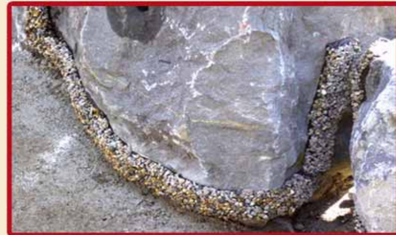
Permanent deformation of a band BFL-Mastix glued on rock.
