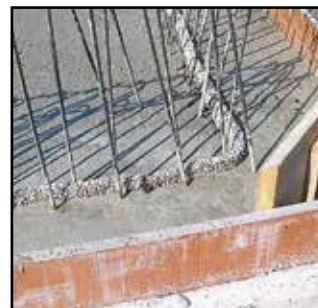
In angles, the bands are bent
