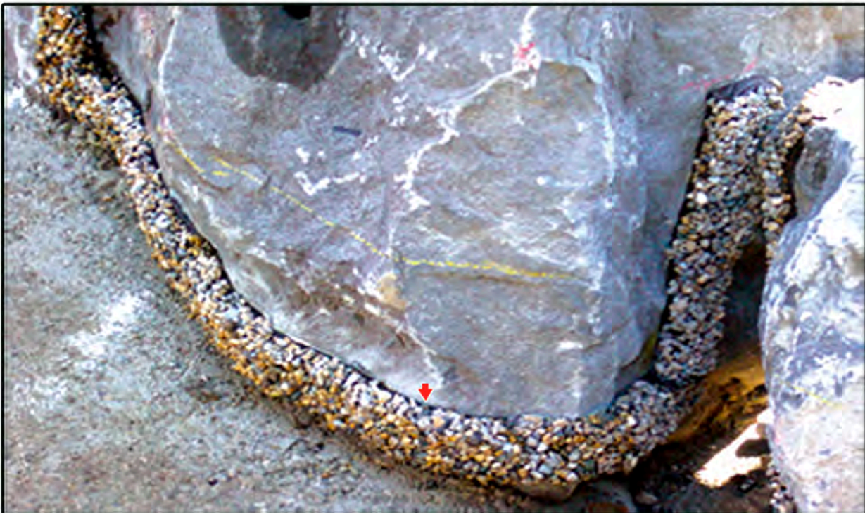
BFL-Mastix bands glued chemically on rock
