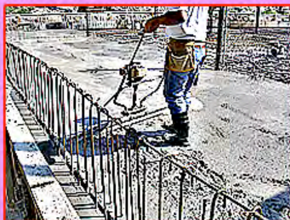
Vibrating after placing the bands
