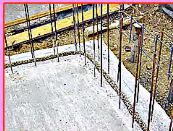
In corners it is possible to bend the bands
