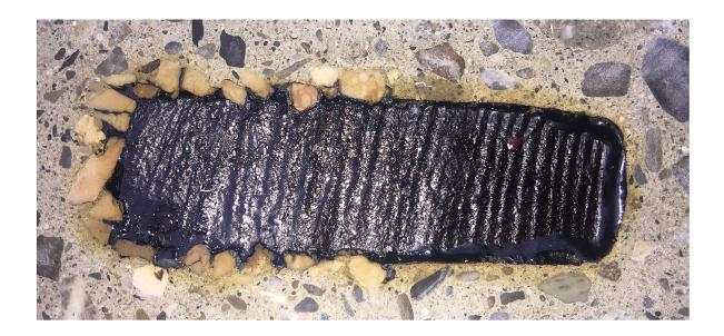
The fine crushed gravel, covering entirely or partly the core of the deformable BFL-Mastix waterstops, assures a perfect physical adhesion with the cement paste in the concrete. This physical adhesion in the concrete is being improved over the years through the chemical adhesion.
