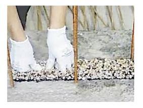
Connecting bands between each other is made with the glue Mastix MS-Polymer. It is necessary to respect, that the glue is not covering the gravel coating.
