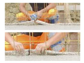
BFL-Mastix waterstops type R4 are incorporated in fresh concrete. Half of their height is in the concrete and half above, in a waiting position.
