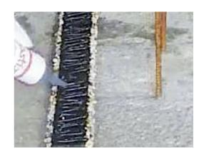
A slight pressure is to be applied on the bands, when glued on the support.
