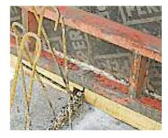
Washing of the work joint surface is done before placing the formwork panels. With wind in summer, the work joint surface must be well moistened in order to avoid the formation of porous spots through a loss of water out of the fresh concrete into the dry raft concrete.
