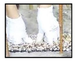
**2** Band connections are made with the glue Mastix MS-Polymer, but without debording on the gravel cover.
